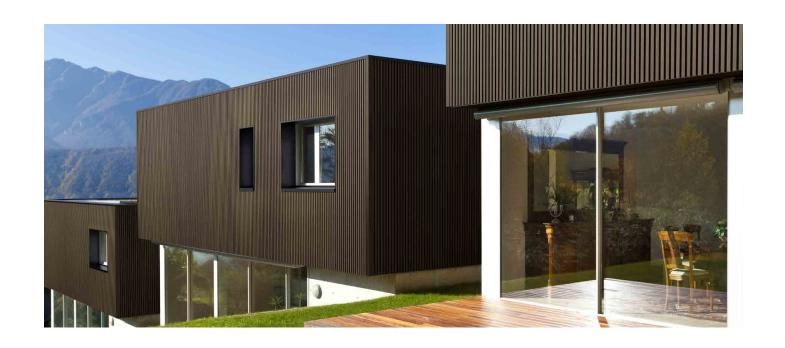
WEO® has a trapezoidal profile for both horizontal and vertical installation
